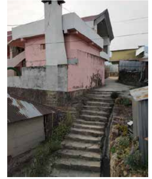
OPEN DRAIN ALONG THE ROAD
